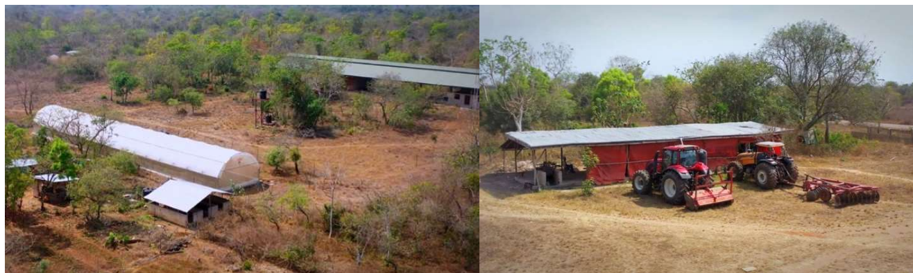
Agricultural Industrial Park expansion (processing center). Two of our tractors prepare to begin work.
